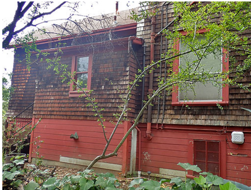
Figure 25. Circa 1940s addition, east façade
