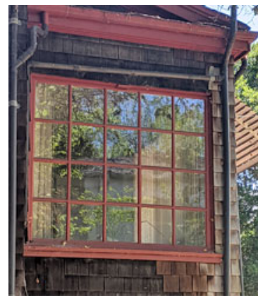
Figure 15. West-facing window in front porch
