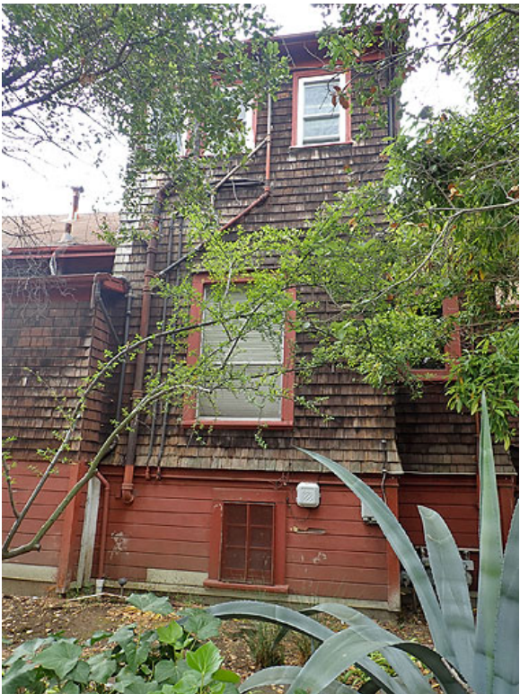
Figure 27. East façade, central section
