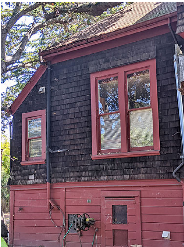
Figure 22. West façade toward the north
