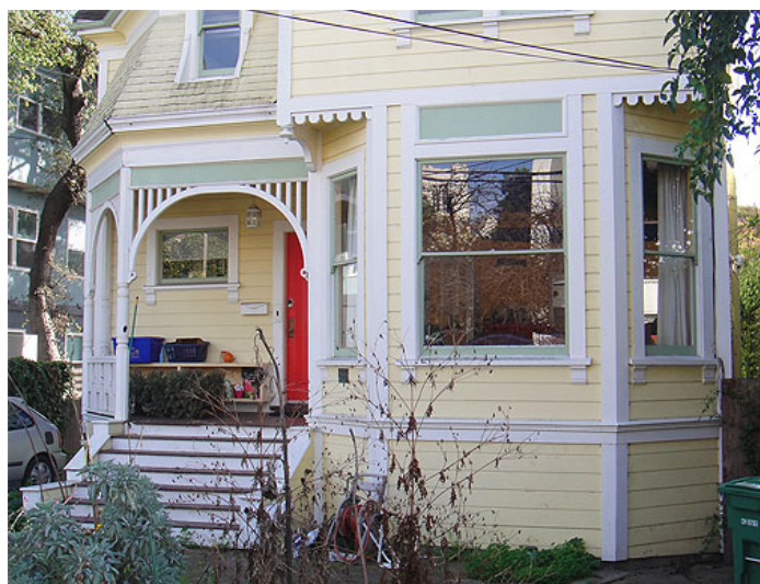
Figure 9. Rustic siding, Luttrell House
