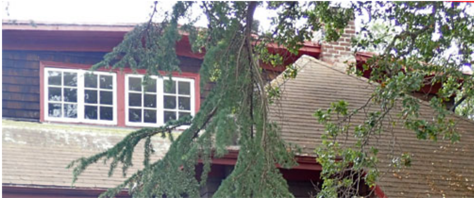
Figure 31. Brick chimney, north side
