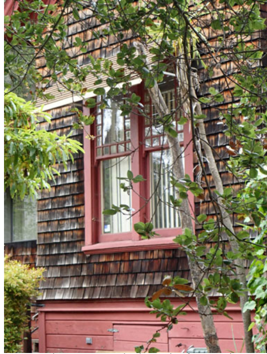
Figure 13. Windows in front wing
