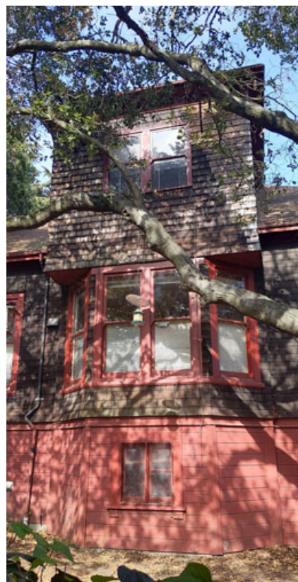
Figure 23. Bay window & second story, west façade
