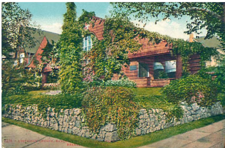
Figure 59. First Unitarian Church (A.C. Schweinfurth, architect, 1898)
