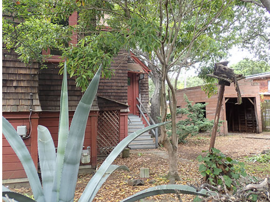
Figure 29. East façade toward the rear & garage
