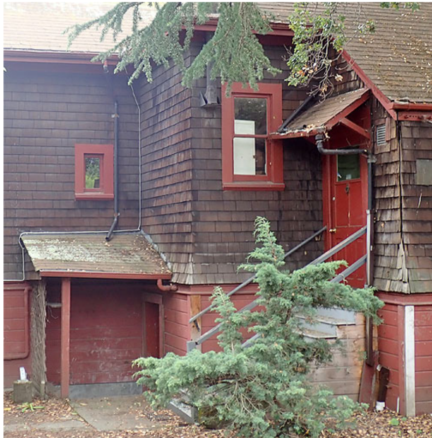
Figure 32. Cellar & service entrances
