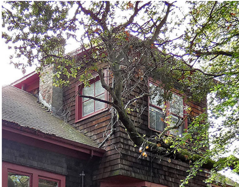
Figure 19. Upper story above west façade
